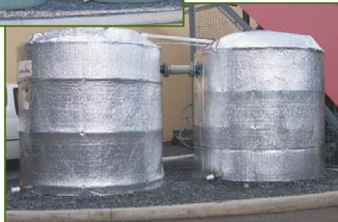
Brine tanks. Before and after insulation
