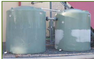
Brine tanks. Before and after insulation
